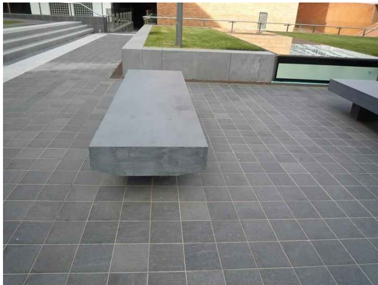
FORMED CONCRETE SEATING
